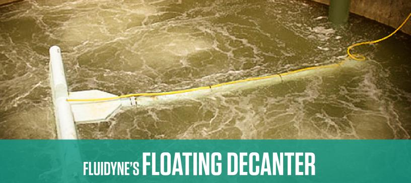
Fluidyne's floating decanter removes supernatant off the top of the tanks in various water and wastewater applications. It is ideal for decanting water from lagoons, digesters, equalization basins, aeration basins and SBRs. The decanter is an all hydraulic design. It floats up and down with changing water levels and can remove liquid levels down to a few feet above the tank floor.
