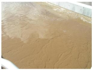
**Excellent Floccing Sludge in Jet MCR**
